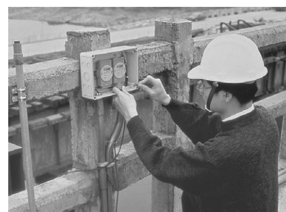
Plug-in Terminal Block Save time by leaving wiring intact while connecting or disconnecting modules
