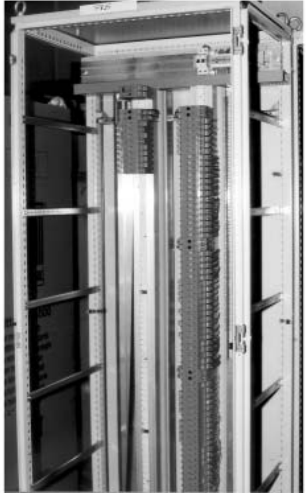
Control cabinet without marshalling
