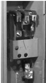
225 A Q-Frame Tenant Circuit Breaker Base (Three-Pole)
