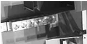
225 A Branch Unit Load Neutral Terminals
