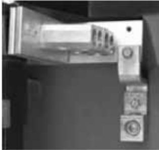
Service Grounding Lug, Bonding Strap, and Bonded Main Neutral Bus as installed on Main Devices at Job Site as Required for use as Service Equipment
