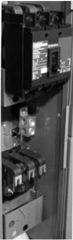
225 A Branch Unit Load Neutral Terminals
