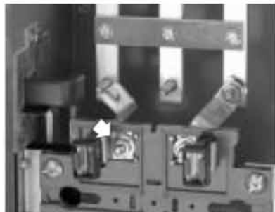
Step 2: Loosen hex nut from AØ line side meter socket jaw and slide "Z" connector down to free connector from stud.
