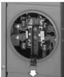
Manual Slider-Type Bypass Shown in Closed Position with Handle Extending through Notch in Rim of Meter Socket Cover
