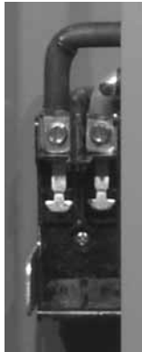
125 A QO Tenant Circuit Breaker Base (Two-Pole)
