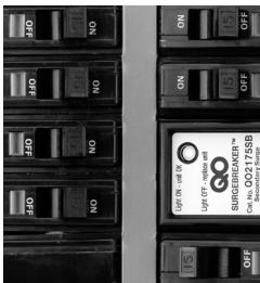
QO2175SB Installed in a QO Load Center
