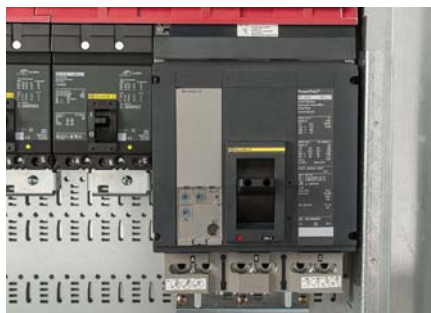
Powerpact P-Frame 1200 A Main
