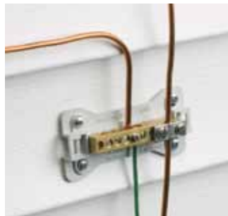
Intersystem Bonding Termination Bar (IBTB)
