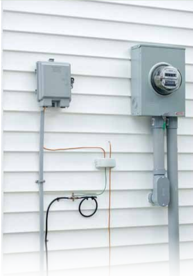
Intersystem Bonding Termination Bar (IBTB)
