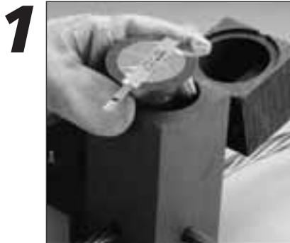
*Insert CADWELD PLUS package into mold (may require use of a cover/baffle)*
