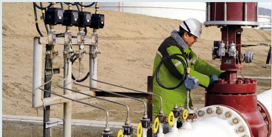
Measurement station sensors on the pipeline
