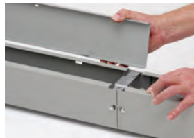
Install and secure hinged covers
