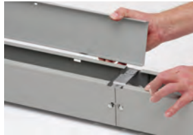
Install and secure hinged covers
