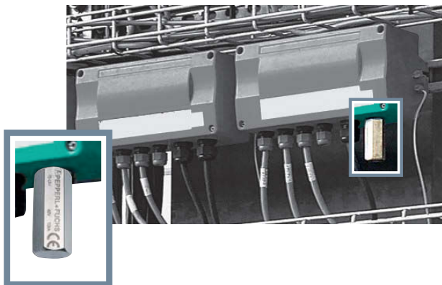
Figure 45 Terminator or surge protector for field installation – the threading can be chosen.
