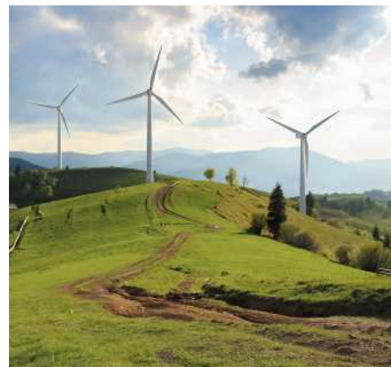
Protected signal circuits at lofty heights
