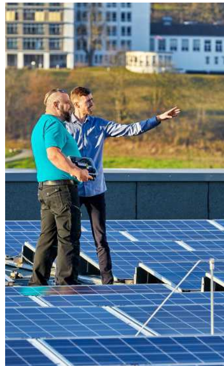
Uninterruptible energy generation
